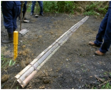
Photo 1: Cross ditch made with stripped Moso bamboo
